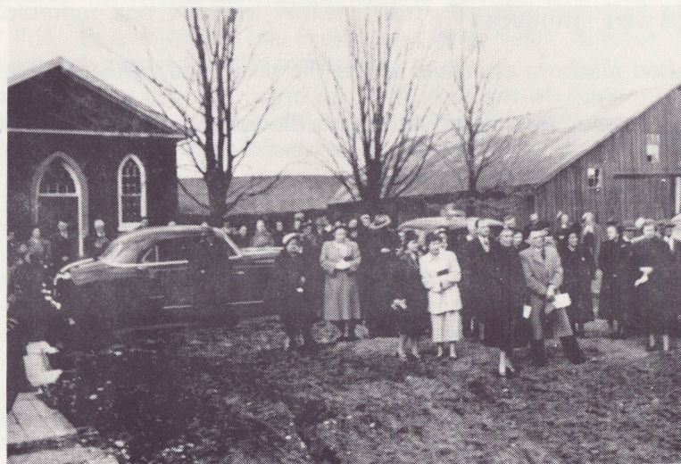
The old church with its two sheds. Picture was taken March 29, 1952, the day the corner-stone of the present church was laid.
