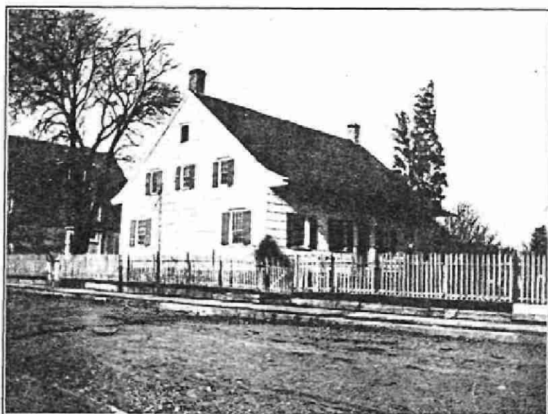
The Old Lake Homestead at Gravesend 12
